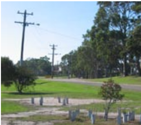
Overhead powerlines on Western Boulevard
